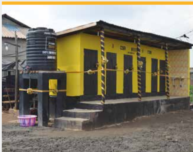
Figure 6: Six new toilets at completion
